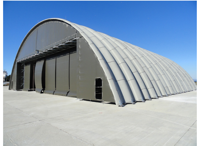
The composite hangar is offered with a range of options, including side covers and access doors.
