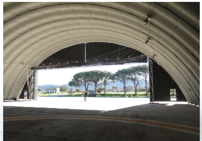
Constructed from prefabricated composite sandwich panels, the Composite Modular Transportable Hangar can be employed in a wide variety of civil or military applications.
