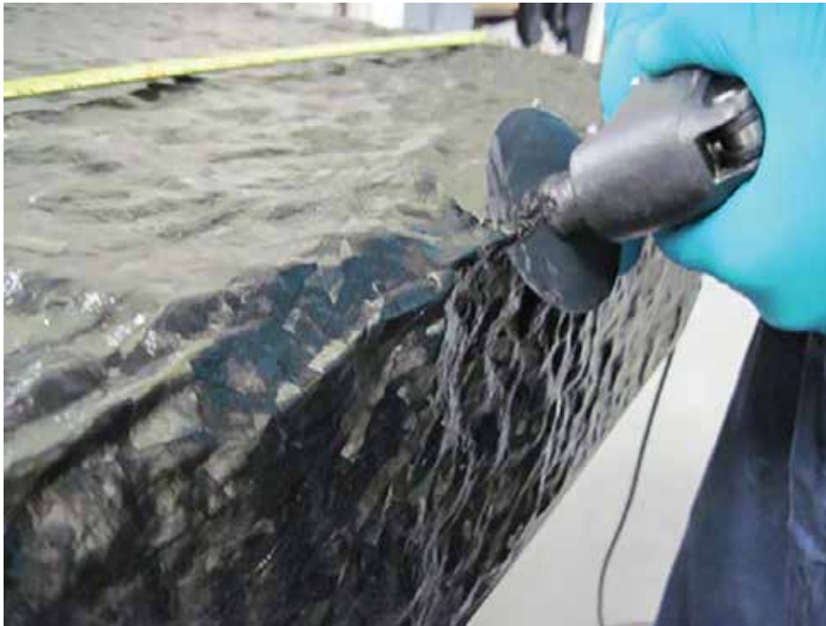
Figure 8: Trimming of high spots or corner pinches/creases with a vibratory saw
